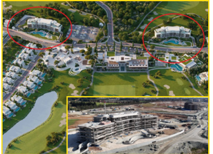
Limassol Green-Robin West and Robin East Residential Buildings - Λεμεσός
